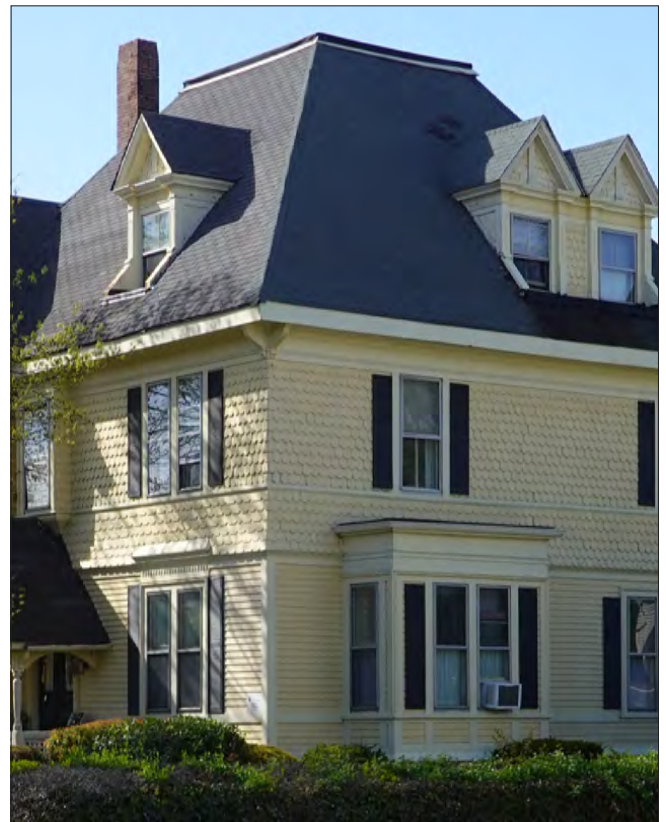
Asphalt is a common replacement material for state or wood shingle roofing.
