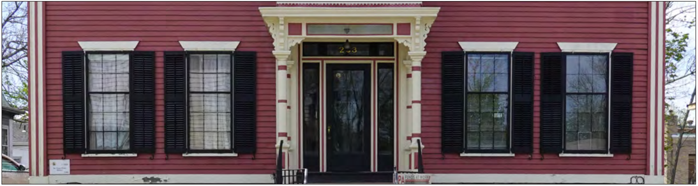
Center-hall homes generally have an door flanked by a pair of windows at each level. In this example, the windows all have 6/9 double-hung sash with wood louvered shutters.
