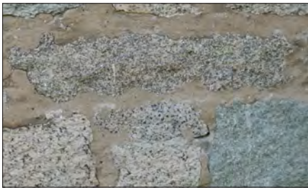
Fieldstone - Locally quarried stone (in this case granite), typically uncoursed of varied sizes, shapes, and colors.
