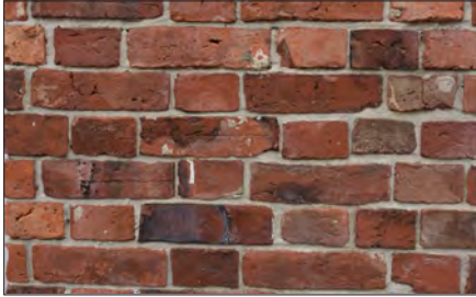
18th-19th Century Brick - A soft, fired-clay, fairly regularly shaped building component; often with color and surface variations
