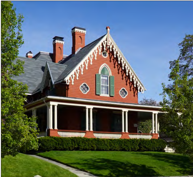
There are a variety of architectural styles represented in Fall River, such as this Gothic Revival residence.
