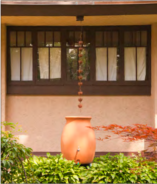
Rain barrels can capture storm water from roofs for use in gardens.
