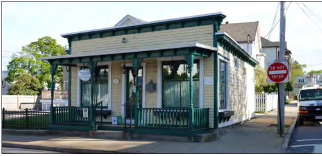
This former store now serves as a medical office.
