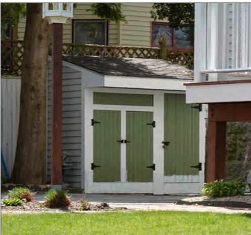
The location of this small structure makes it minimally visible from the public right-of-way.
