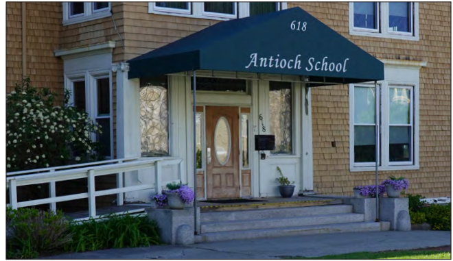
The accessible ramp allows all visitors to enter through the same door while maintaining the stair configuration.
