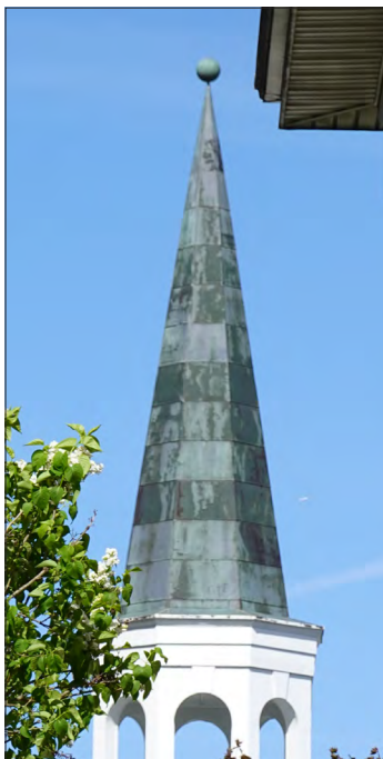
This copper, flat seam metal roofing is formed from pieces of metal that are joined along a seam and soldered together.
