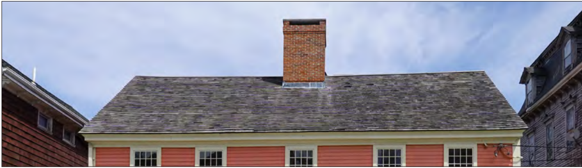
Massive central chimneys are often found at Fall River's oldest buildings.
