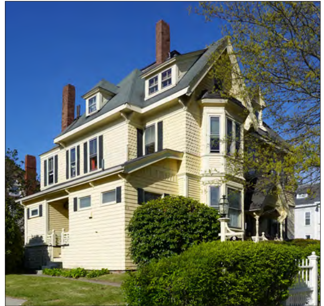
The side elevation addition is subordinate to and compatible with this residence.
