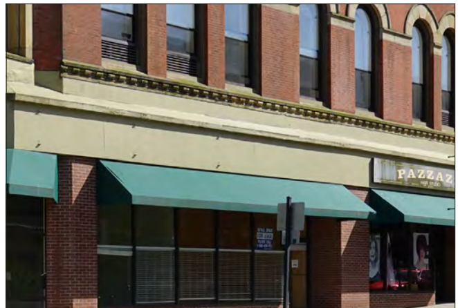
Storefront cornices can be highly decorative and serve to separate the storefront from the building above.
