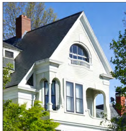
This eclectic residence includes asymmetrical inset porches at the second floor and a small balcony at the third floor, visually relieving the otherwise flat facade.
