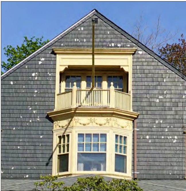
The projecting, second floor oriel window provides a third floor balcony accessed by a central door. This two-story feature provides a visual focus for an otherwise simple elevation.
