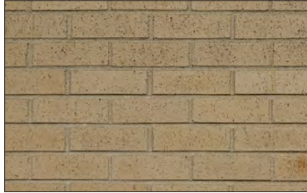
20th Century Brick - A hard, dense, fired-clay, regularly shaped building component; sometimes glazed.
