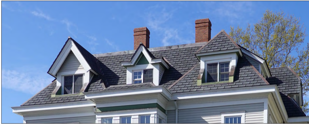
This house features three dormer windows with different roof forms: a standard gable, a gable with flared eaves, and a dormer with a hipped roof. Also note two prominent brick chimneys.
