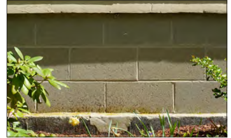
Cast Stone Units - Formed masonry units made from water, cement, and sand aggregate.
