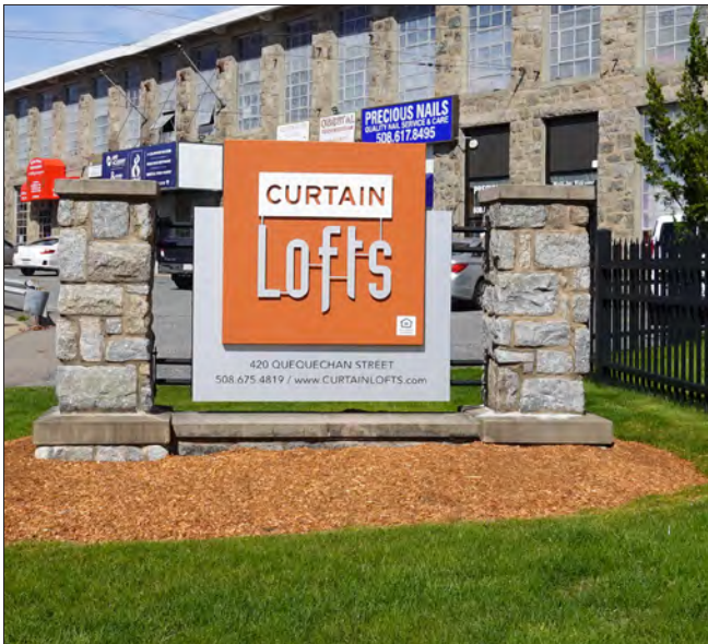
The granite piers supporting this freestanding sign complements the wall material of the historic mill building.
