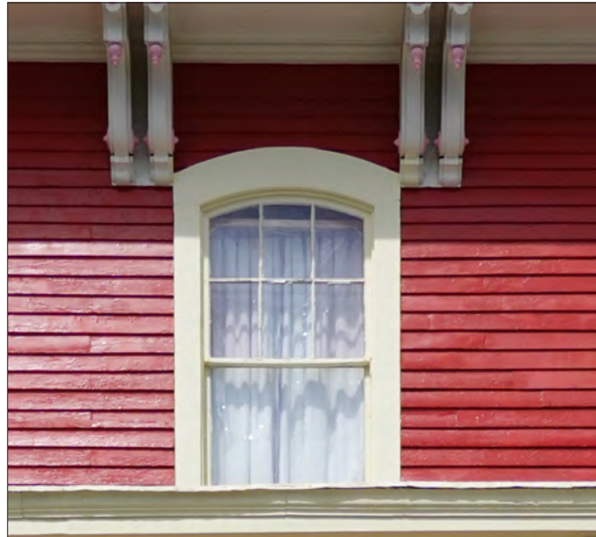
Arched-top windows are often found at Italiante buildings, which also feature decorative cornice brackets.
