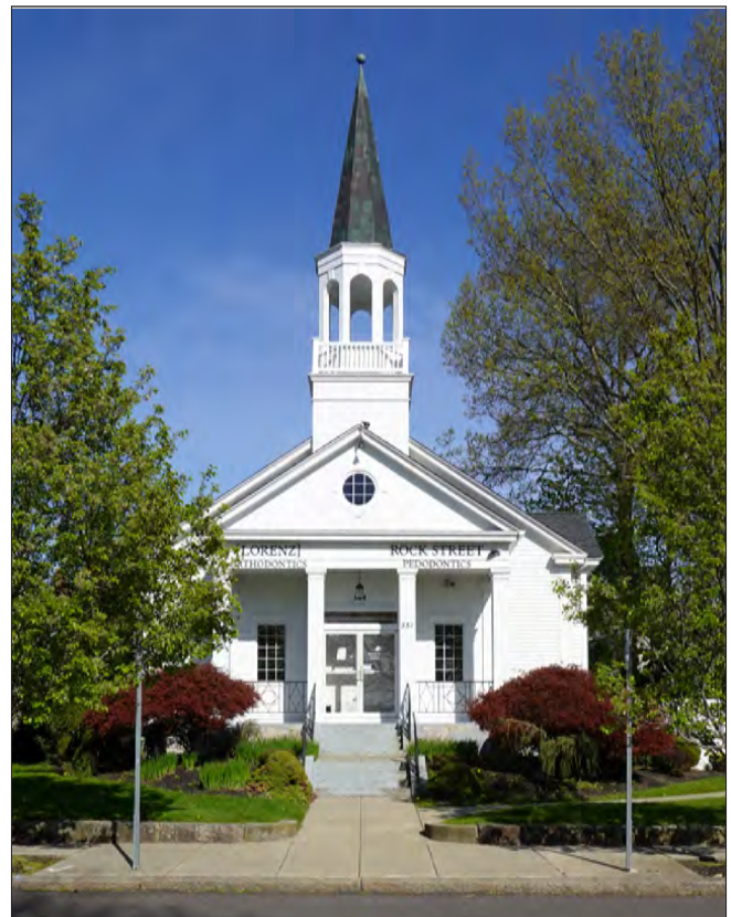
This former church now serves as a medical office building. By renovating and adaptively reusing the existing building, a significant local structure was saved from demolition and the current office has a unique and easily identifiable location.
